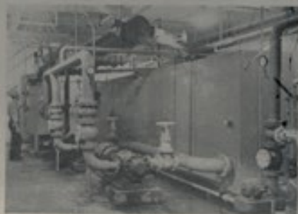
This oil circulating system pumps 250 gals. a minute
